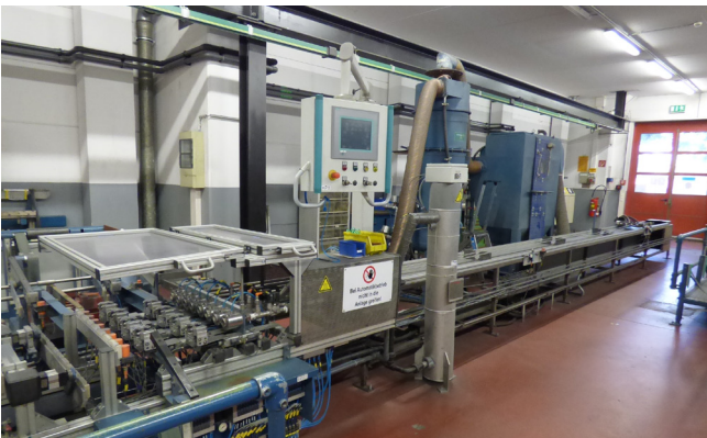
Pos. 257 1 Rohr-Innensandstrahlanlage AREVA, Bj. 1996/2009 1 Tube interior sandblasting system AREVA, YOM 1996/2009
