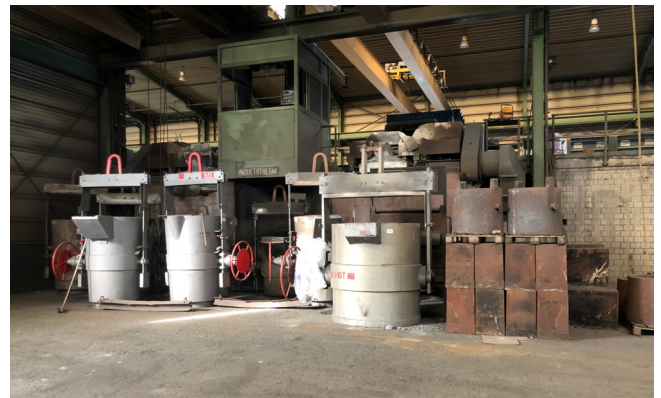
Pos. 4 1 MF-Induktionsofen-Anlage, Bj. 2007 1 MF Induction melting furnace system, YOM 2007
