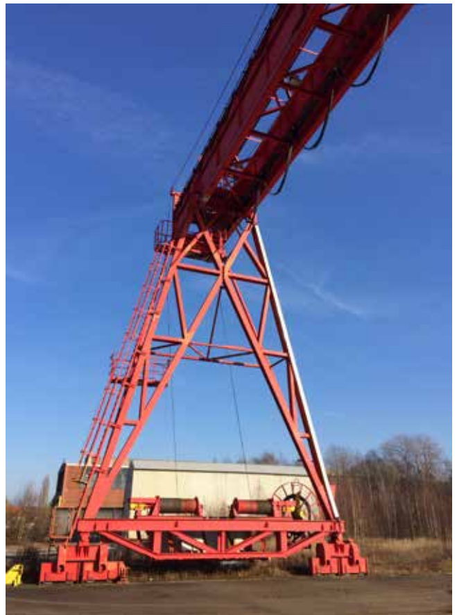
Pos. 774 1 Portalkran 1 Gantry Crane
